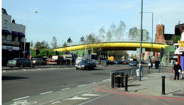
The Green Bridge
