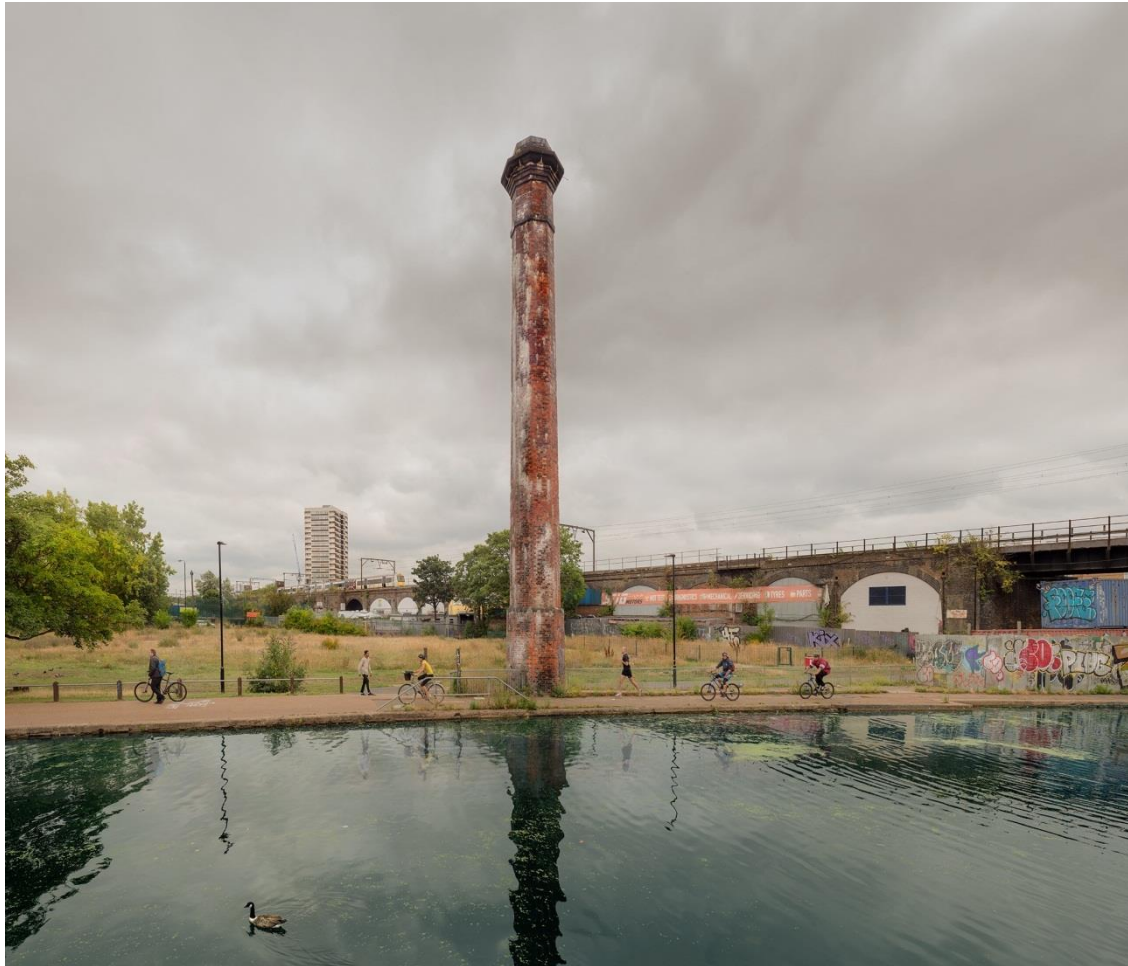
Brick Sewer Ventilation Shaft in Kirk's Place
